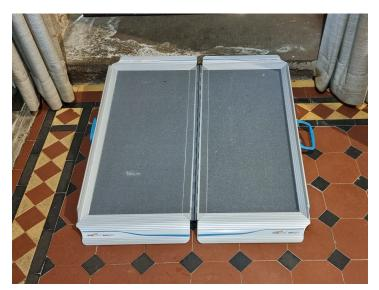
The inside of this threshold step has a 10cm drop to the tiled floor and a metal portable folding ramp is available for wheelchair users. Otherwise the floor of the nave and aisles is tiled and level.
